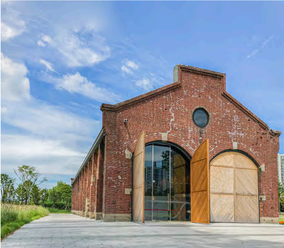
Vehicle Maintenance Depot at Jinju Station
